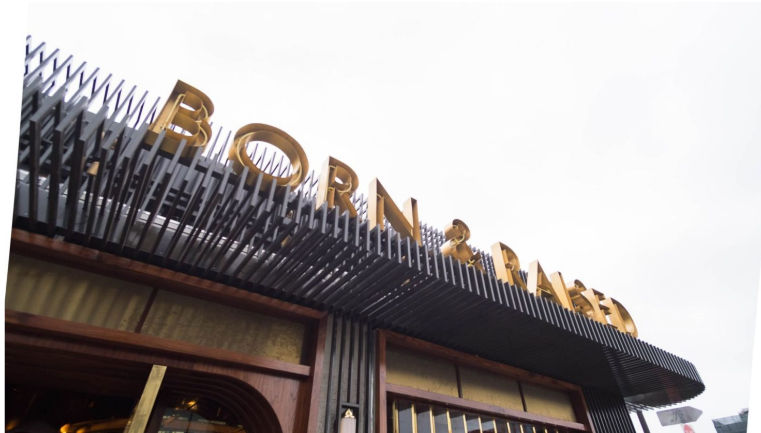
METAL VERTICAL DETAIL @ FRONT FACE OF BULDING C/W SIGNAGE INSTALLATION CONCEPT
